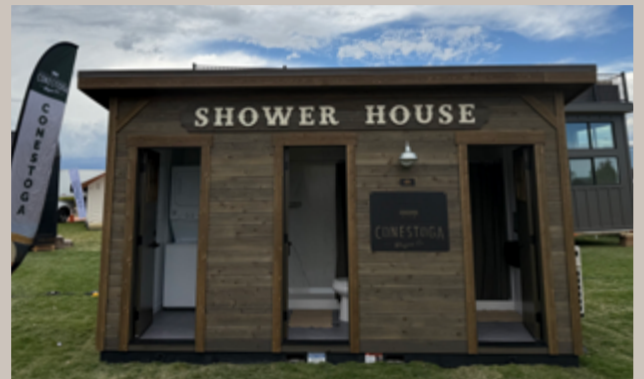
3-ROOM CEDAR PANELING SHOWER HOUSE
